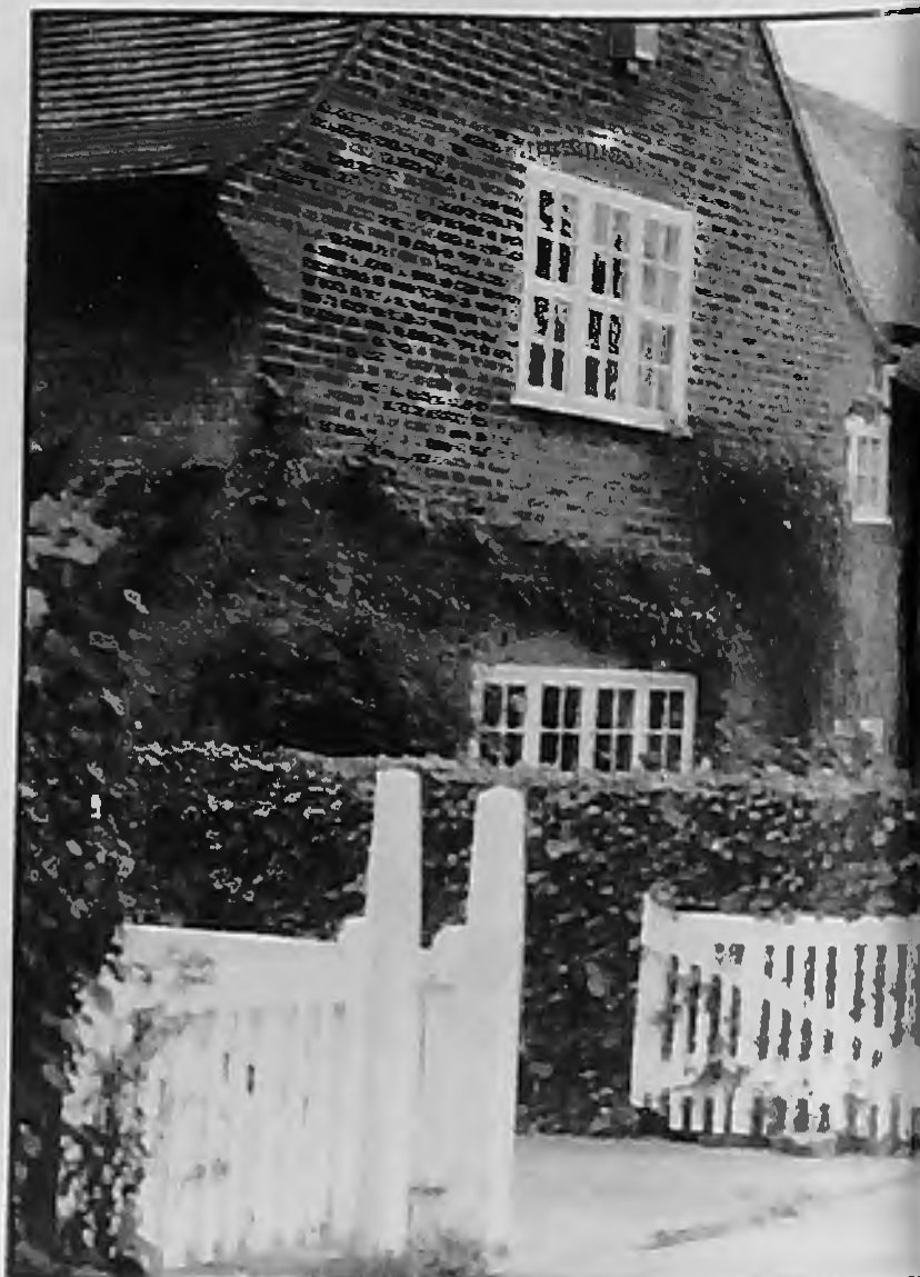
A photographic Survey of the Garden
