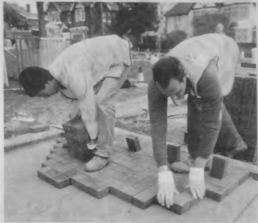
Work began at the beginning of March on the Friary Environmental Zone traffic management programme. This includes traffic calming, cycle routes, road junction improvements and width restrictions.
