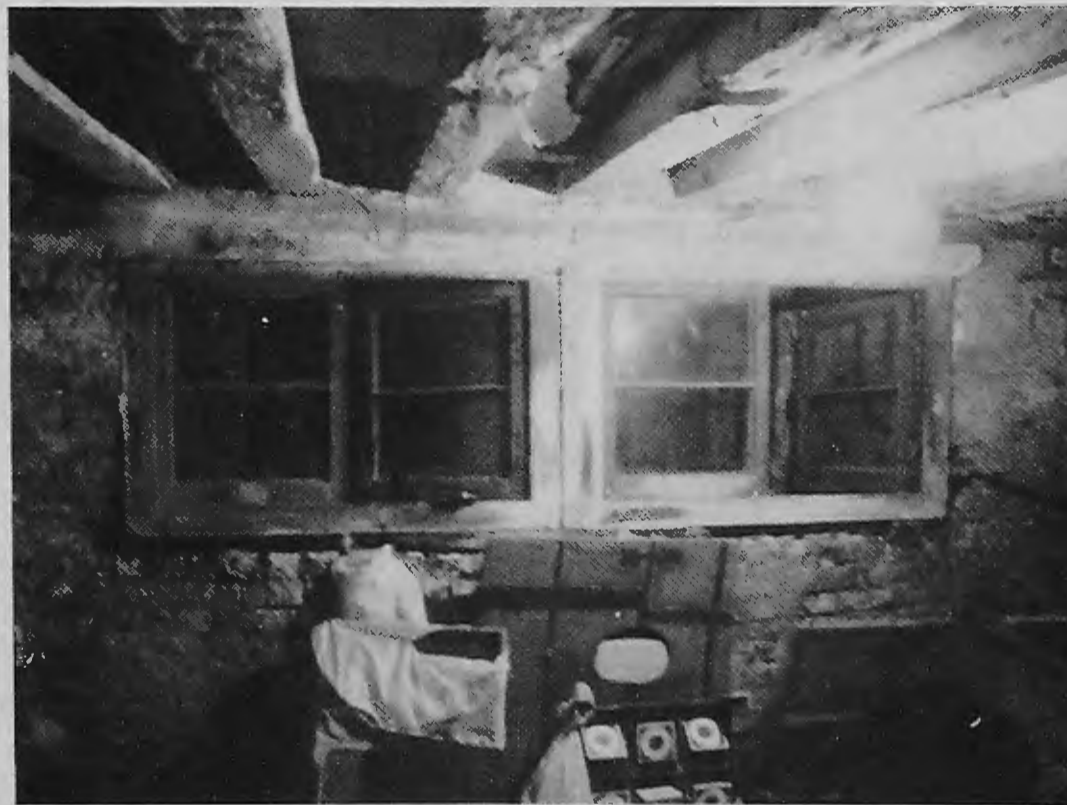
The cellar has original floor joints and antique window.
