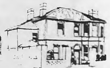
PREPARATORY DEPARTMENT (ST. ALBANS) Woodside Lane N12
