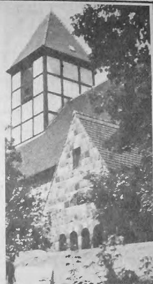
Parish Church of Tempelhof.
