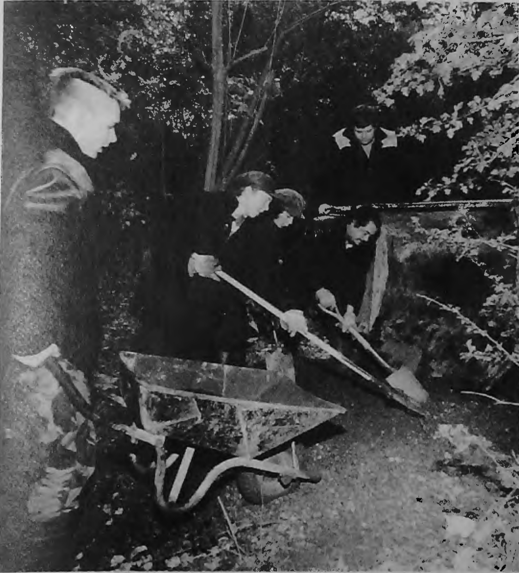
Working on the Page Street Line — shovels and rakes at the ready as road planings are tipped to make a surface. Left to right, Ben Crowley, Melissa Bainbridge, Sally Triteos and John Bryan with a little overhead supervision from Ian Faulkner.
