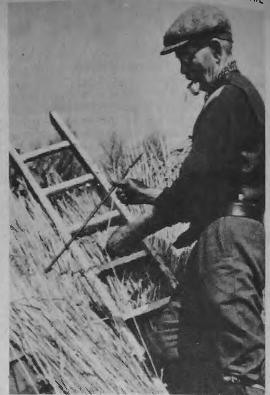
Thatching the roof during the restoration of Church Farm House, 1954.
