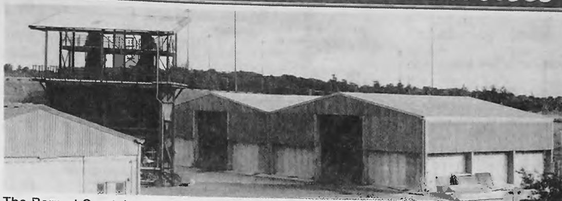
The Barn at Scratchwood to store salt and keep it dry to avoid wastage.
