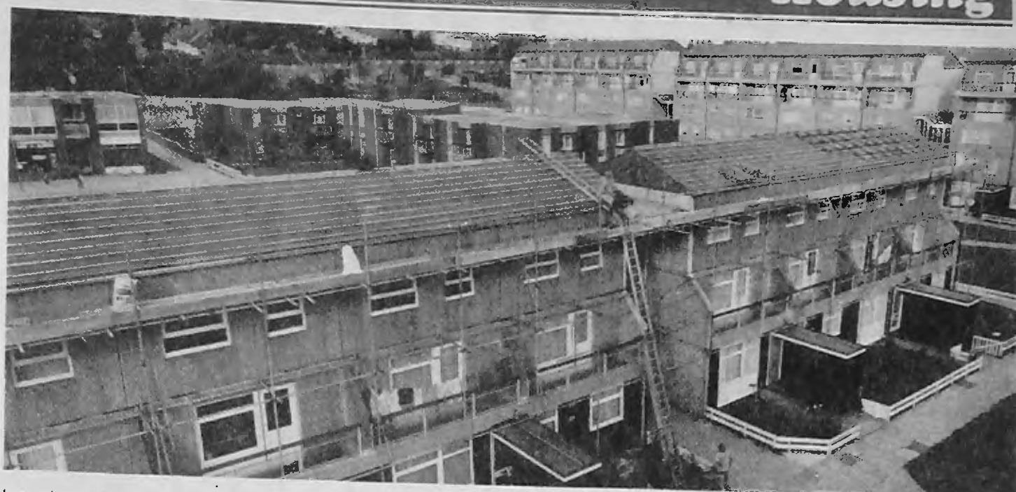
New pitched roofs being built on the flats at Dollis Valley.
