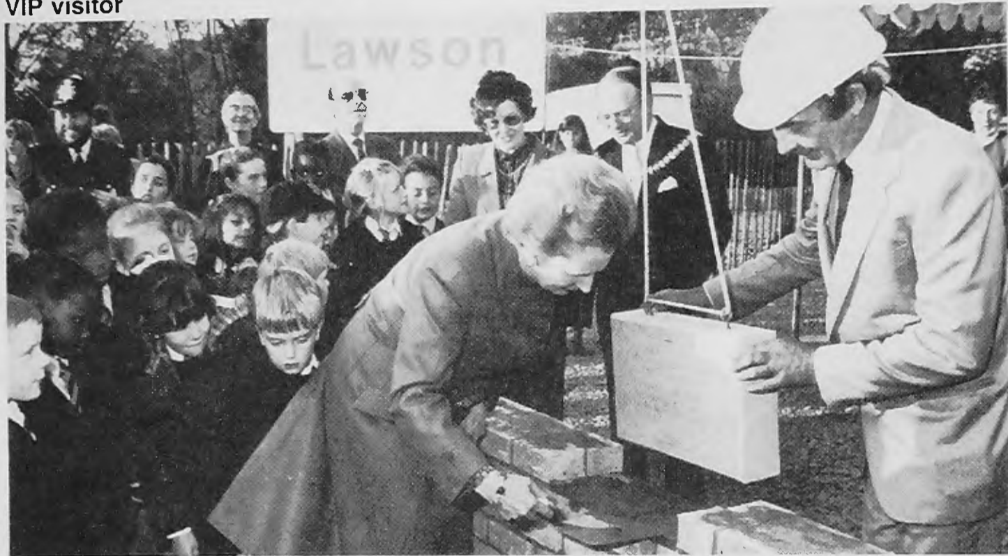
The Prime Minister, Mrs Margaret Thatcher, MP for Finchley, lays the foundation stone of the new St. Mary's C of E Junior School with a little help from Tony Henry, site manager for Lawsons, the contractors
