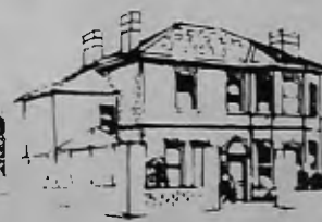
PREPARATORY DEPARTMENT (ST. ALBANS) Woodside Lane N12
