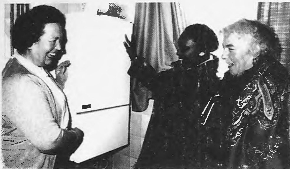
June Withey shows ward councillors Agnes Slocombe and Doreen Neall (right) the new boiler
