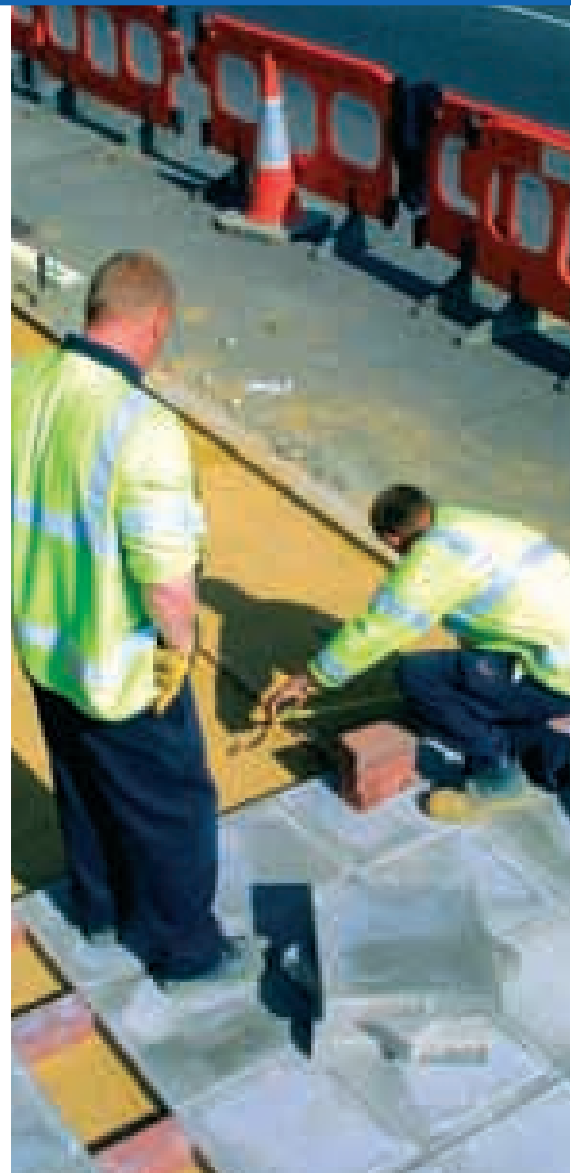
Improvement work being undertaken in Barnet
