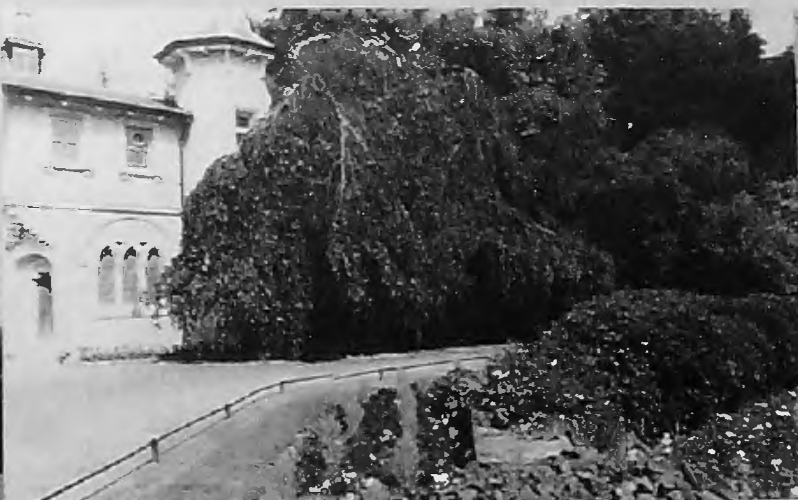
AVENUE HOUSE, GROUND, FINCHLEY
