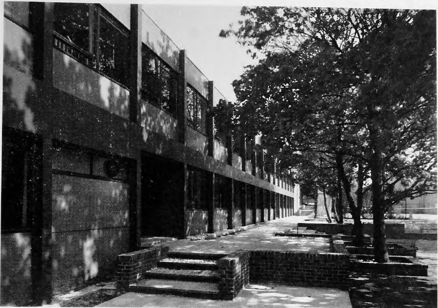
The main elevation of the Fern building
