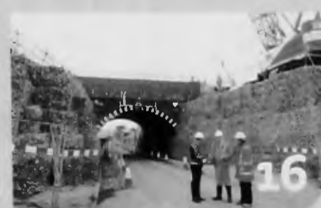
16 New bridge project
