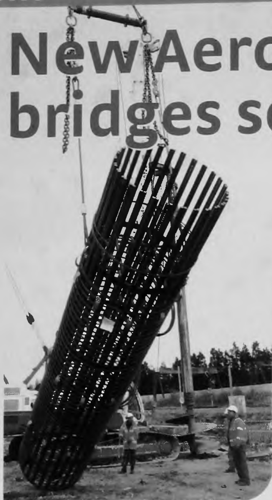
Work to modernise the bridges begins at the site in Colindale
