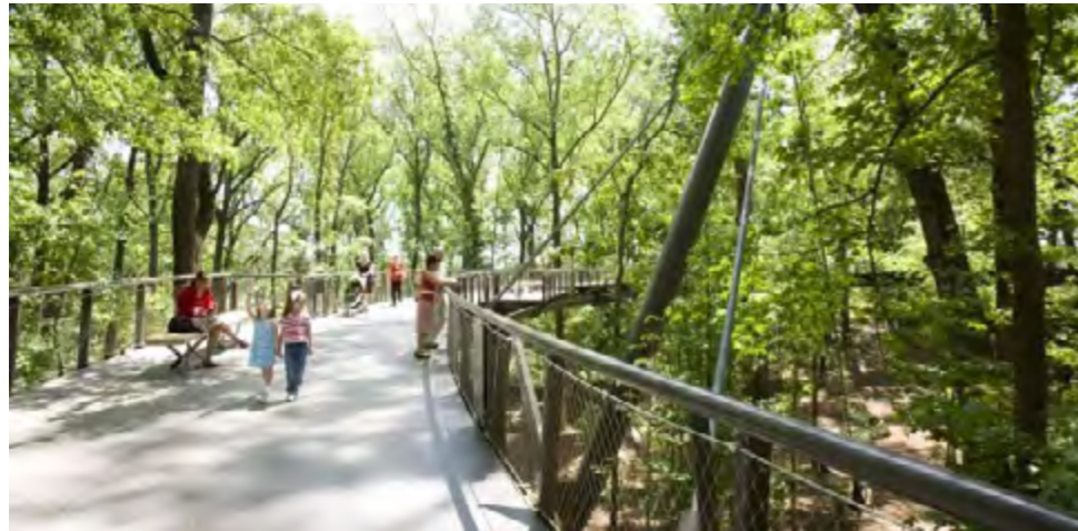
Flyover pedestrian bridge
